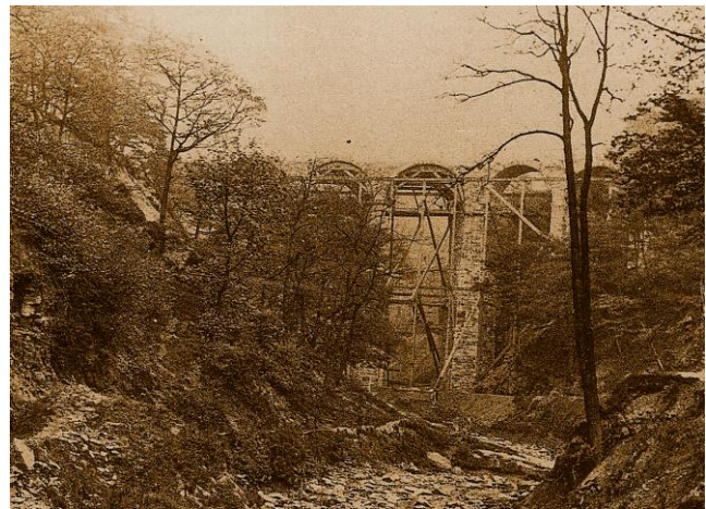
Healey Dell Viaduct under construction around 1866. From An Illustrated History of Rochdale's Railways , J. Wells, 1993.
