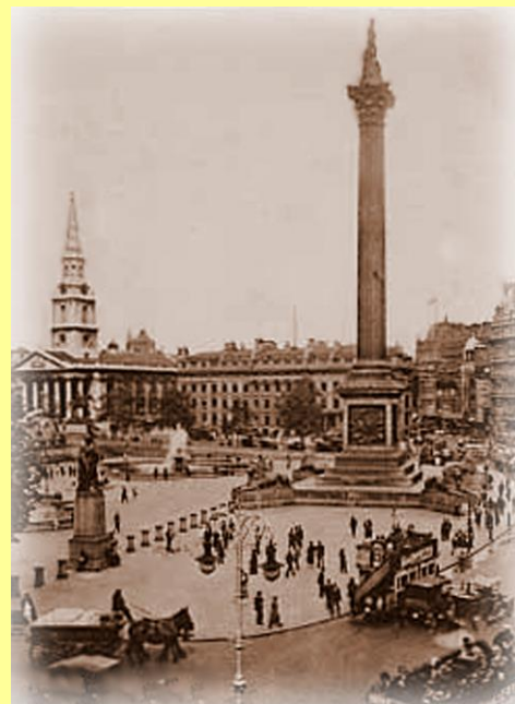
Locally it is claimed that locally quarried stone that was finished at this mill was used in the building of Trafalgar Square in London!
